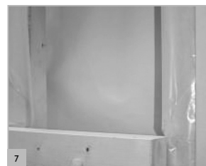
7 Install the wooden surround for Ignis-Protect into the studwork.
