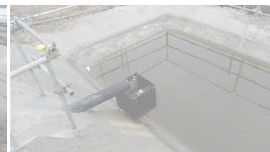
The final discharge through a Smart Sponge® Ultra Urban Filter was tested by the EA.
