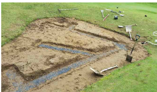
Marking out installation (10.00 am)
