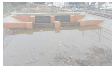
The completed Enviroflow filtration scheme showing all 3 stages of treatment
