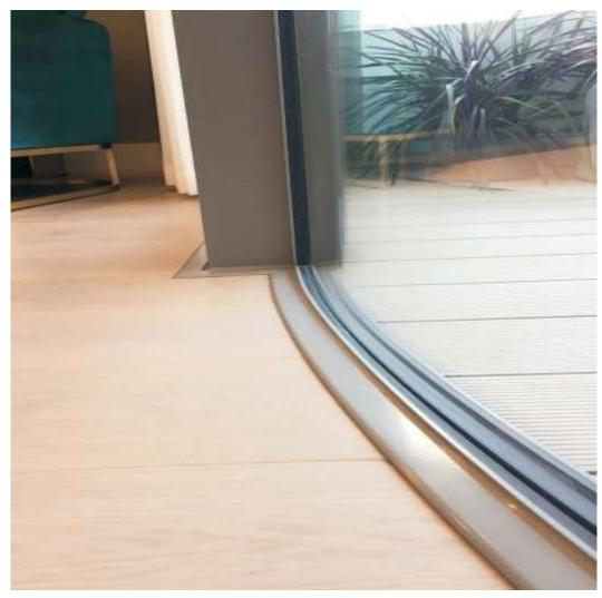
Perimeter Detail: Kliks End Stop curved to radius of balcony doors. Powder coated to facade RAL colour. Seamlessly allowing expansion.
