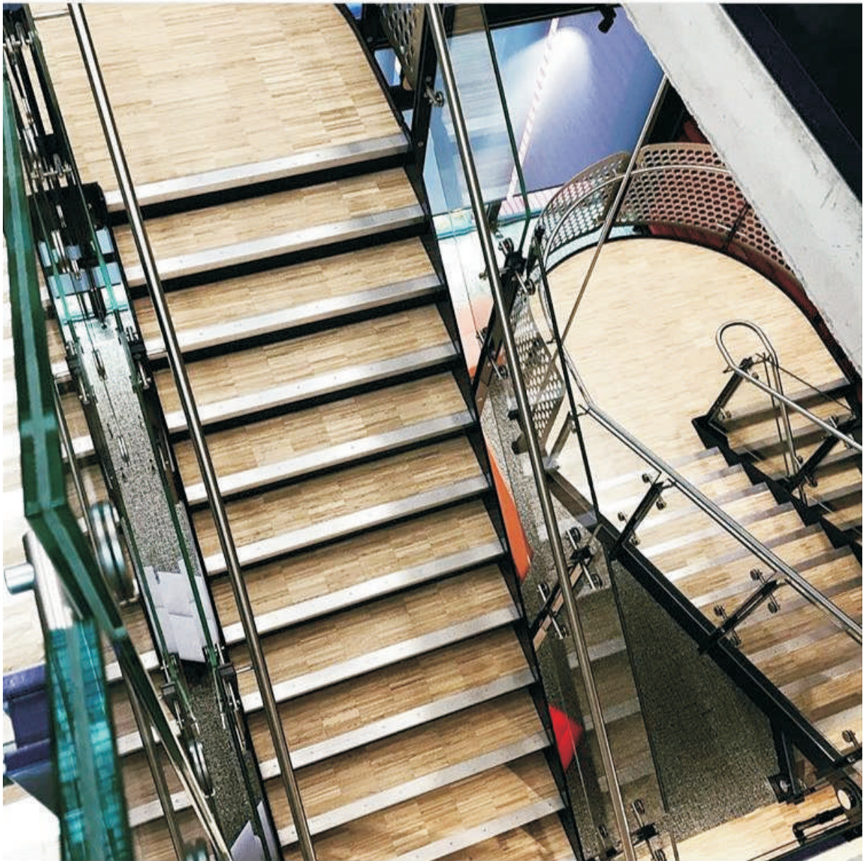
AN6R castellated aluminium stair nosing installed into TFL Building, London. photo credit Loughton Contracts
