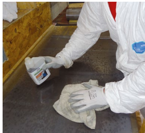
Patentation oil to the lead flashing
