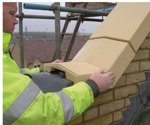
Clip on pre-mitred sections and stop ends as necessary.
