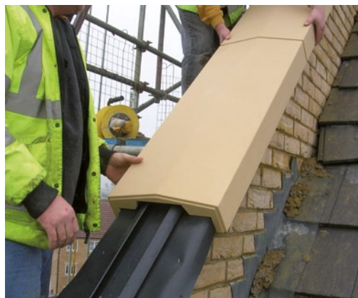
Simple clip system to fix copings in place easily.
