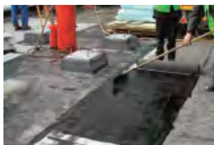
Install final layer with protection sheet.
