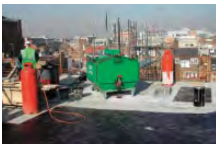
Apply Radmat Surface Conditioner
