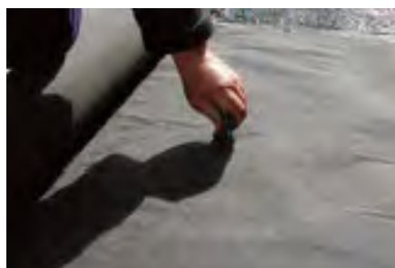
Check thickness of system.
