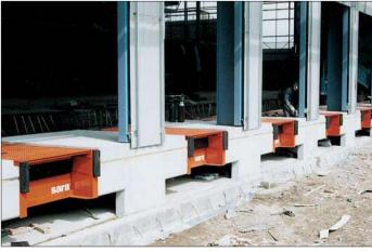
sara Levellers being set in sara Pre-cast Concrete Pits
