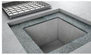
**Step 4:** Lay a mortar bed of minimum 40mm thickness all around the shaft opening the full width of the frame.
