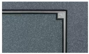
**Step 9:** Refit the cover and check there is an even gap between the cover and frame. Insert all locking screws and hand tighten to securely lock the cover. Refit all locking screw dust caps. Once the materials have fully cured, the access cover is now ready for use and service loads. Retain all spare parts, the installation and maintenance booklet and lifting/locking keys for future use.
