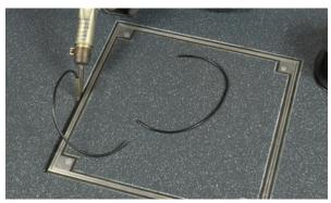
**Step 8:** Once the final floor has been fully installed, remove any excess adhesive or grout from around the cover and frame. Open the cover with the lfting/locking keys provided. Clean all surfaces and ensure the sealing areas of the cover and rubber seals are free from debris. Lubricate all seals with a suitable silicone grease.
