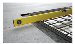
**Step 5:** Bed and level to the access cover and frame centrally over the shaft opening ensuring the top edges of the access cover and frame are at the finished vinyl floor level. When tapping down to level use a piece of wood to protect the upper surfaces. Ensure the frame is fully supported by the mortar with no voids. Allow mortar to sufficiently harden.
