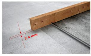
**Step 6:** Ensure the reinforcement provided is placed at the bottom of the cover. Haunch the frame fully with concrete (min 150mm wide) and fully fill the cover to within 2-4mm of its upper surface to suit the thickness of vinyl flooring to be installed. Vibrate concrete where necessary to ensure no voids and the weldable PVC trim is fully supported.
