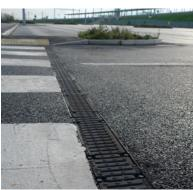
To support a wide variety of catchment depths, hydraulic capacities and applications, the system is available in four channel widths and is offered in constant and sloping depths for optimum performance and system design.
