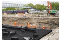
The open cell structure permits completely free access for CCTV and jetting equipment which allows the whole system, including all the extremities, to be inspected and maintained from just a few access points.
