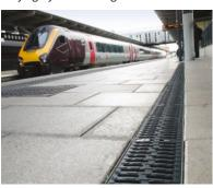
To provide a wider choice of products, an alternative base is available. ACO MultiDrain PPD is a high strength channel drainage system manufactured from recycled polypropylene.
