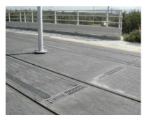
ACO TramDrain 200 is manufactured from Vienite®, ACO's sustainable high strength material. The material does not absorb water therefore does not conduct electricity and will provide protection against stray current.
