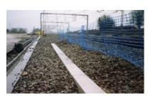
Manufactured from Vienite, ACO's sustainable high strength material, the cable trough is resistant to mould, frost and UV attack.
