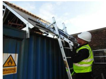
Slide the roof ladder up and over the Lower ladder onto the glazing bars.
