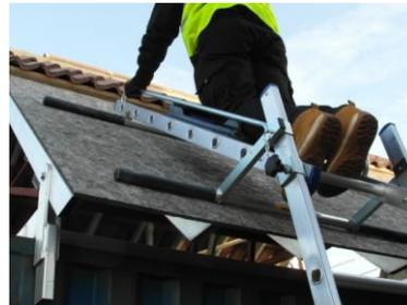
Slide the kneeler to desired position on the roof ladders.
