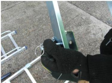
Remove the pins from the Eaves batten.
