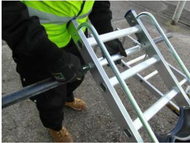
Attach the top batten to the roof Ladder section using the captivated pins in the holes of the stiles. Ensure the pins are pressed home fully.
