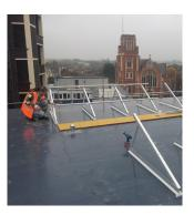
2. Flat Roof Triangles fitted to ICB Solafix and mounting rails attached
