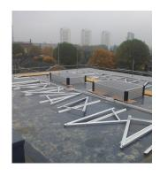
**1.** ICB Solafix System pre welded to the roof, PV Panels lifted & Flat Roof Triangles assembled on-site
