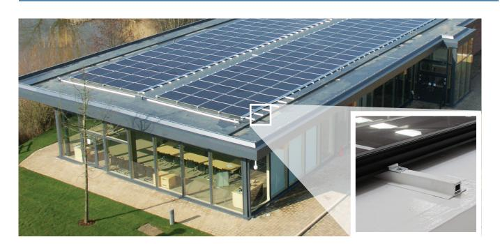
The ultra-light ICB - SOLAFIX fixing system makes it possible to attach solar panels onto the roof without the need for extra ballast or perforation of the roofing membrane. The development of the system has taken into account the abilities of EVA roofing membranes to have compatible elements welded directly to them. The method will allow a variety of different solar panels to be installed quickly and cost effectively.
