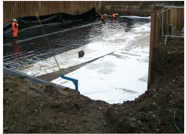
Geotextile membrane being laid
