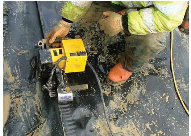
Geotextiles being welded
