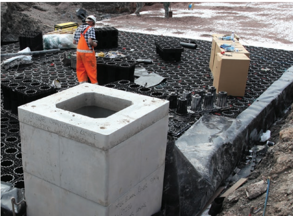
Installation of ACO StormBrixx with Man access units
