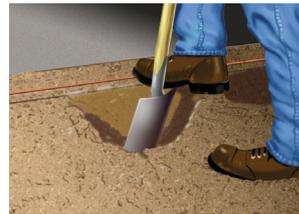
Dig trench, allowing for width of channel plus 100mm each side for concrete haunch. Trench depth should allow for channel depth plus 100mm for concrete bedding. Also allow for 100mm concrete around and beneath sump unit. Mark finishing height with fixed line 3mm below final surface. Lay 100mm (min) bed of concrete.
