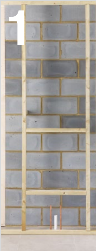
01 Install timber frame (supplied by others).
