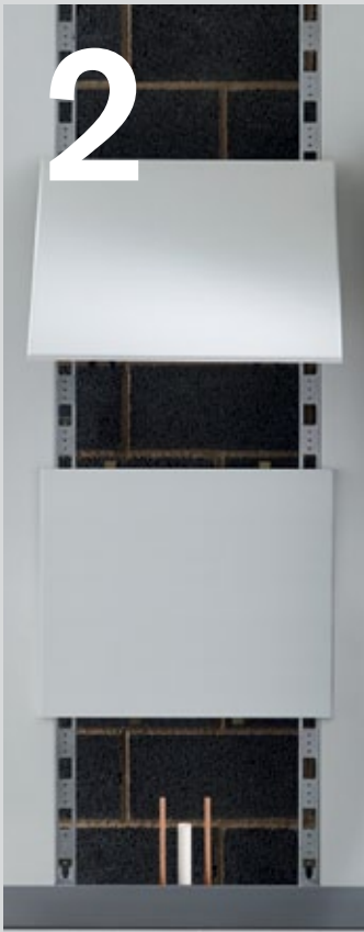
02 Click-fix the first Frameduct unit onto the frame and slide into position. Open the mid panel to a fully hinged position. Attach a vertical flashgap to the frame, on either side of the unit, screw-fixing to the frame from the face. Fix tie back to the wall. Repeat until all units are in place.
