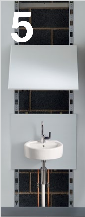
05 Once all the units are in position, connect the plumbing and services and apply silicone sealant to sanitaryware.
