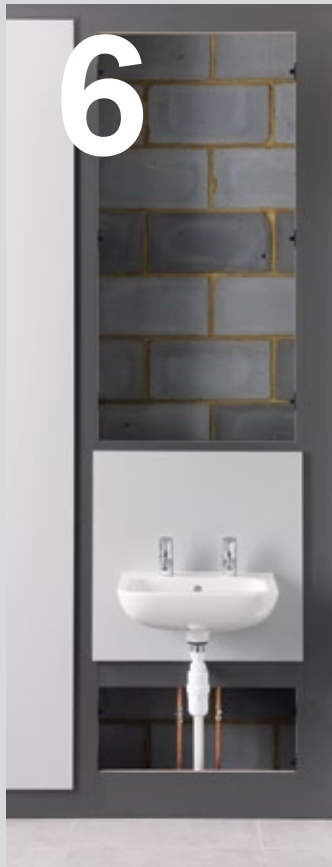
06 Once all the units are in position, connect the plumbing and services.
