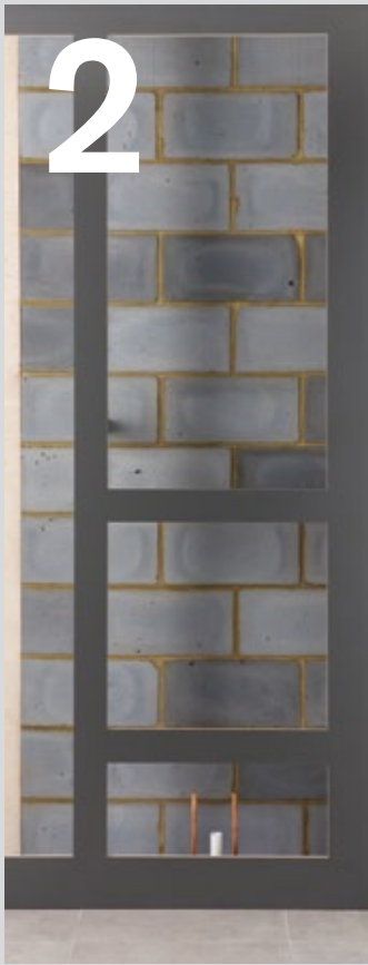
02 Fit base flashgaps to the site frame followed by vertical, horizontal and top flashgaps.
