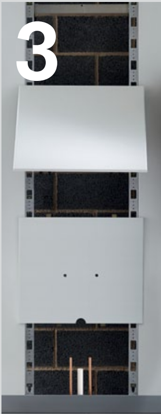
03 Drill or cut out for sanitaryware.
