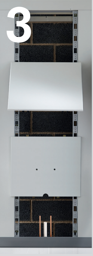
03 Drill or cut out for sanitaryware.
