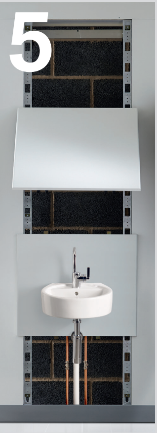
05 Once all the units are in position, connect the plumbing and services and apply silicone sealant to sanitaryware.
