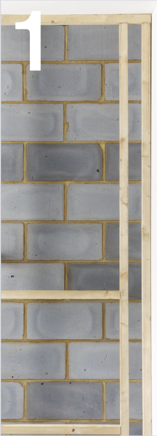
01 Install timber-frame (supplied by others).
