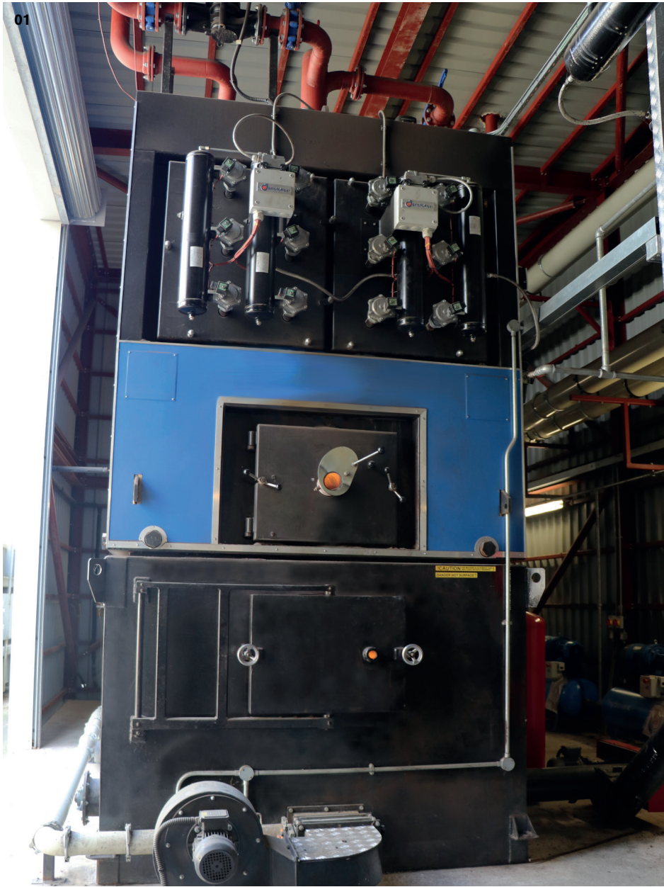
01-02 Waste management Biomass burner turns production waste into factory and office heating.
