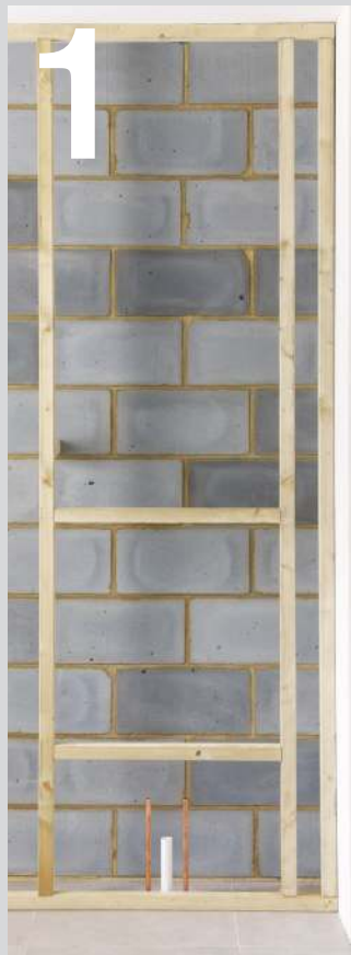
01 Install timber-frame (supplied by others).
