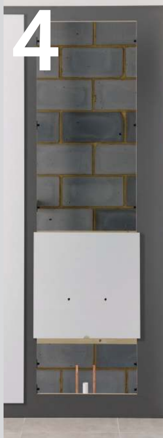
04 Drill or cut out for sanitaryware.
