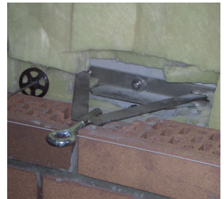
HALFEN HGA-Q Scaffold anchors with short ring bolt. The side struts absorb loads parallel to the façade.
