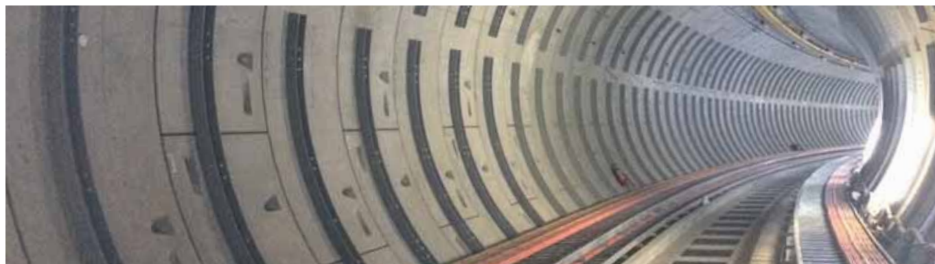
Singapore Power Transmission Cable Tunnel Project – HB-BZ
