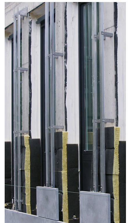
HALFEN UKB Channel support structure
