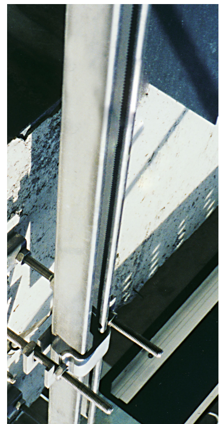
HALFEN SUK Channel support structure
