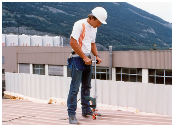
Fixing trapezoidal sheet metal using self-tapping screws
