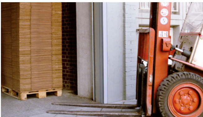
Corner guards in an industrial environment
