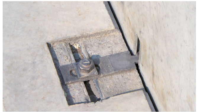
HALFEN HKZ Restraint tie with serrated washer
