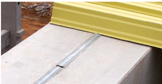
Fixing of trapezoidal metal sheeting roof element
