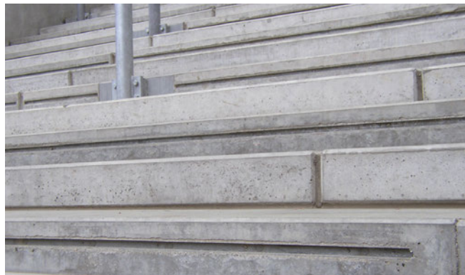
Fixing of safety rails, Rheinenergiestadion Cologne
