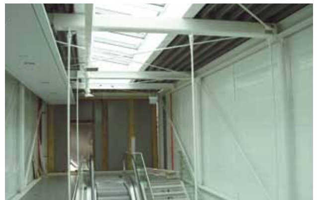
Suspension and bracing of the stair-well structure.
