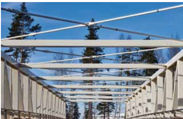
Horizontal bracing of the lattice framework.
