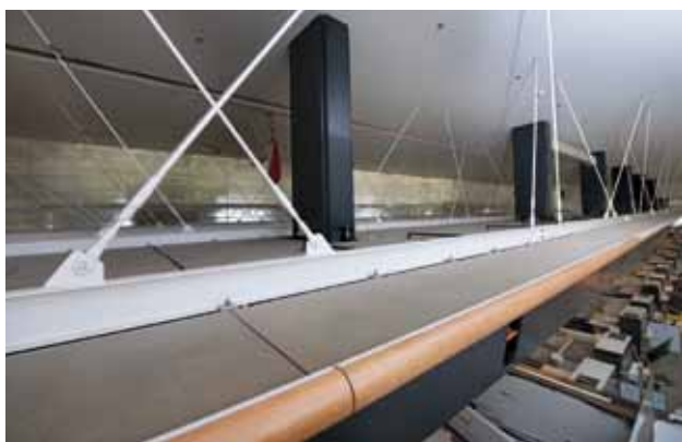
Bracing a suspended installation.
