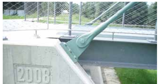
Connection flange with fork-head.
