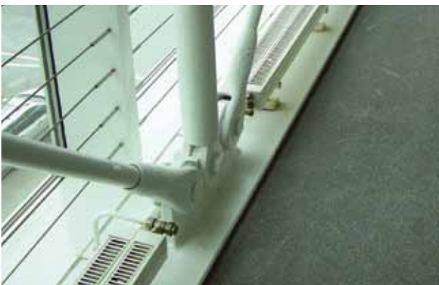
Connection node with welded flange and fork-head; with a white-paint coating.
