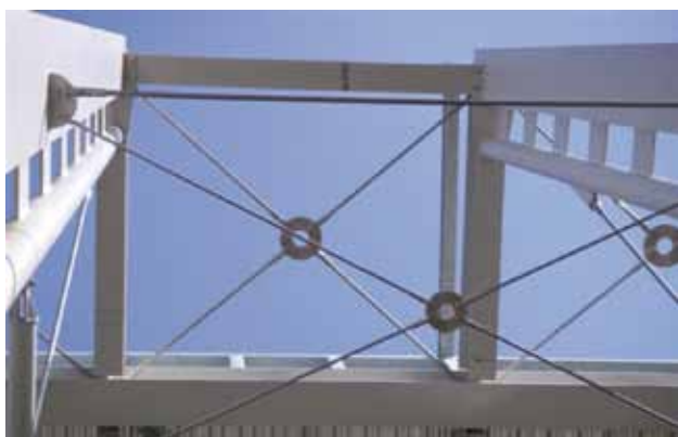
Horizontal and vertical bracing with anchor disc couplers.
