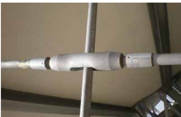
Safe and aesthetic pleasing connection with cross-coupler, counter-nuts and tension rods (during installation).
