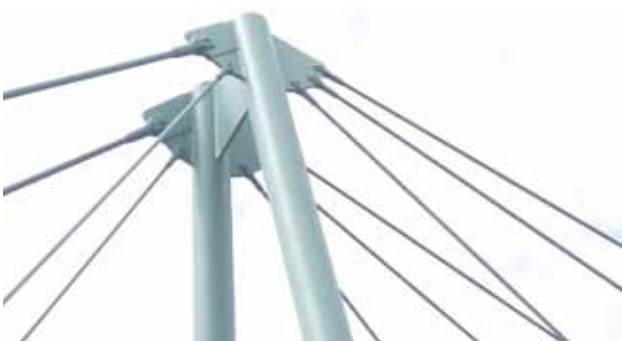
Aesthetic connection of 2 and 3 filigree fork-heads to the support structure.
