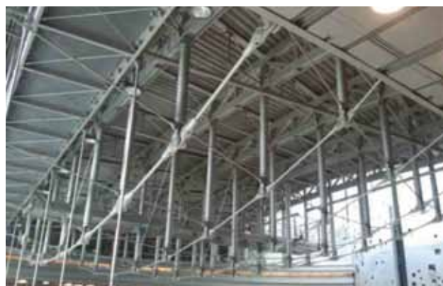
Aesthetically pleasing tensioning and bracing of the roof elements.
