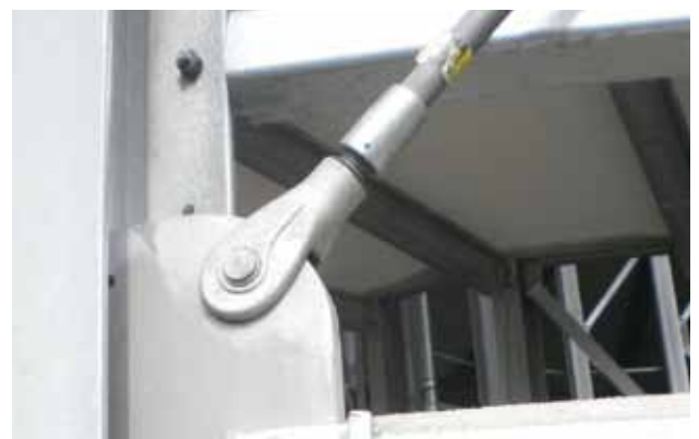
Fork-head (during installation) as connection element.
