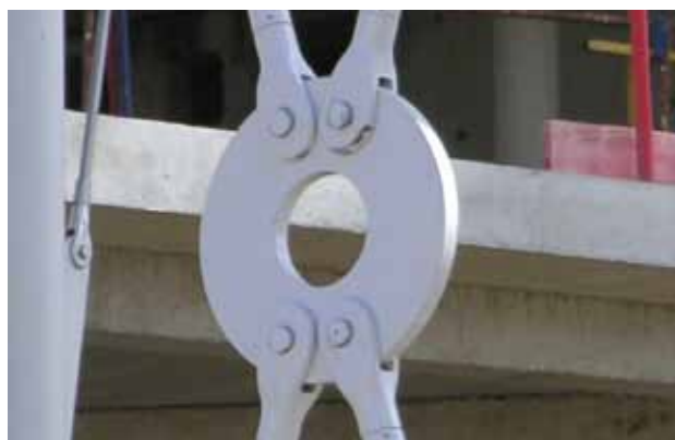
The protective coating (duplex-coating) can have two purposes: architectural design using colour and increasing the corrosion protection.
