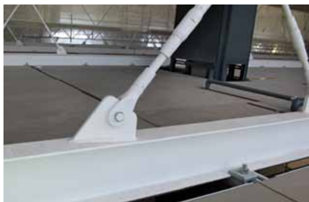
Fork-head with coupler to adjust the system length.
