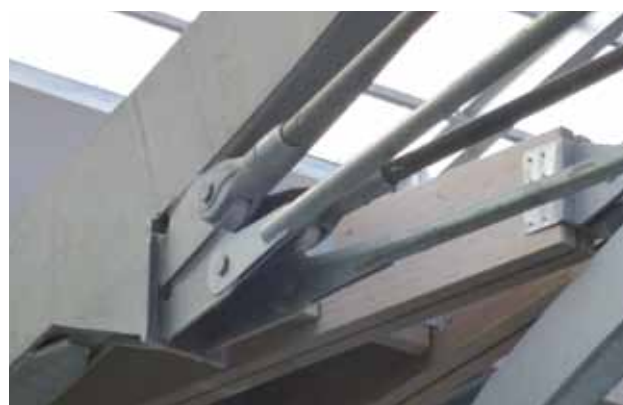
Connection with flange, fork-head and tension rod.
