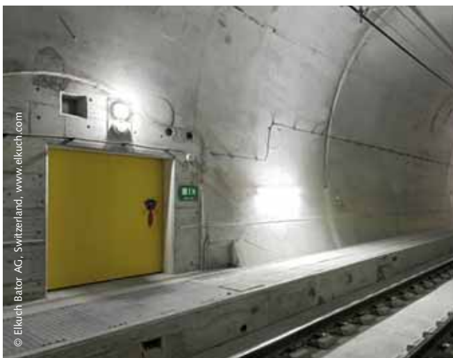
Cross passage door, closed, Lötschberg Base Tunnel
