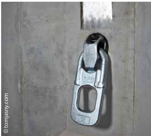
Wall recess with accident recovery anchor and clutch
