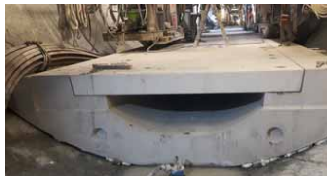
Cross section showing the base segment in detail with cover slab in place
