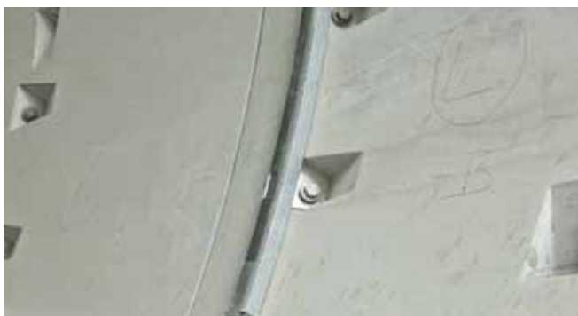
HM 72/48 Framing channel bolted to transverse joint
