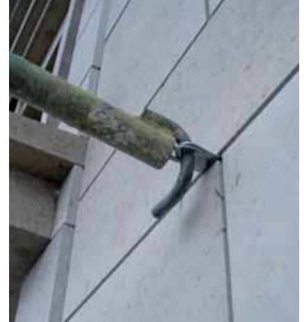
Scaffold element connected to a strap
