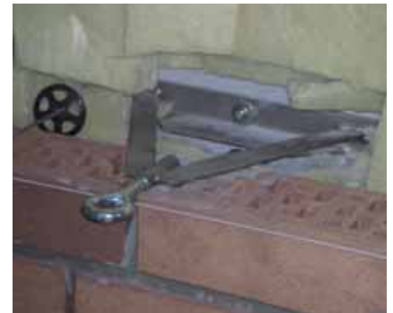
HALFEN HGA-Q Scaffold anchors with short ring bolt. The side struts absorb loads parallel to the façade.
