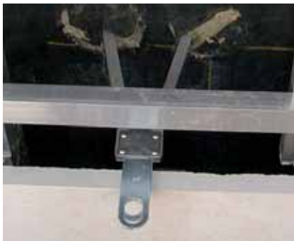
HALFEN GE-HB Scaffold anchors for natural stone façades
