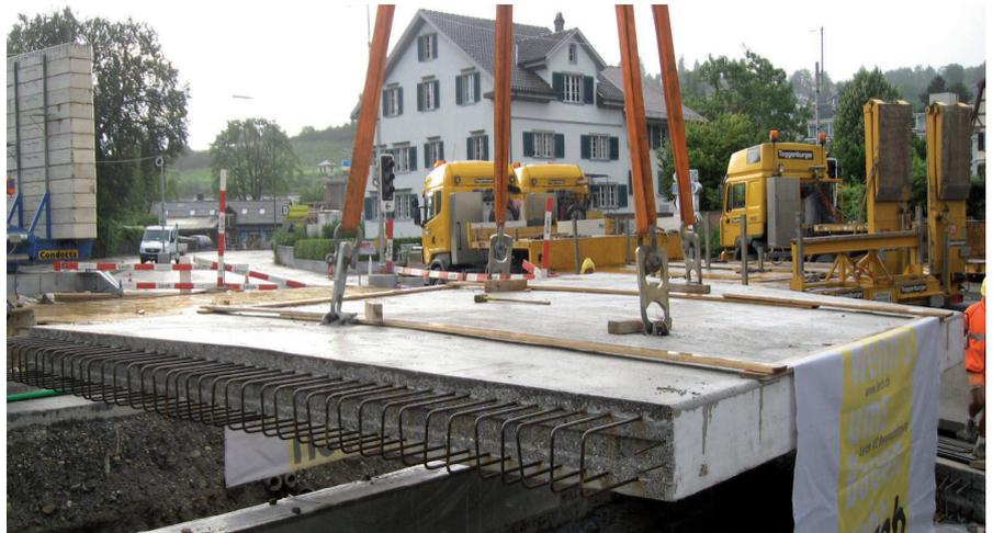
It is inevitable that elements sometimes need to be manoeuvred over critical areas and facilities. The failure of an anchor here can have devastating consequences. Even with correct calculation, deviant material quality can still constitute the critical weak spot. Anchors are subject to further stress especially from dynamic loads (shock factors). Impact strength and elongation at failure are both critical here. Selecting high quality raw material is therefore of the uppermost importance.
