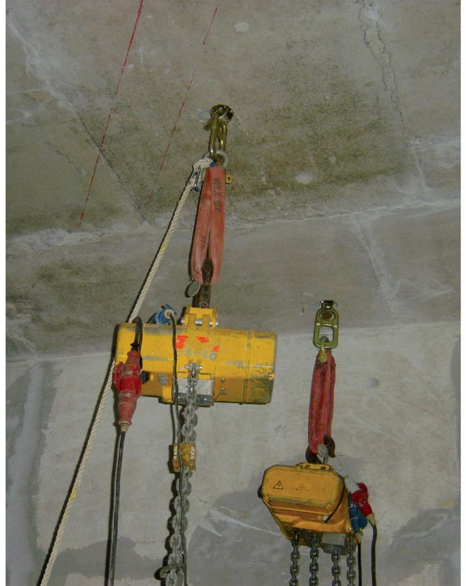
Lifting anchors can be cast in to the roof to facilitate installation and to secure heavy equipment for maintenance. A universal lifting head is attached for installation. A chain or cable is passed through the attached link. The universal lifting head link has a hole through which a safety clip can be inserted (safety clips available as a standard item). This ensures the link is held securely in place.
