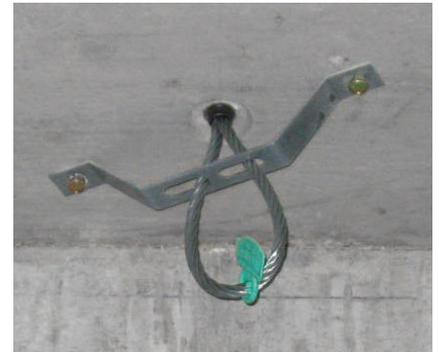
Cable loop installed in a lift shaft
