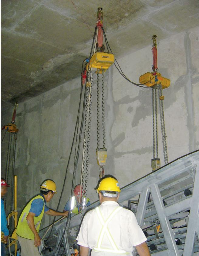
Typical setup for an overhead anchor system
