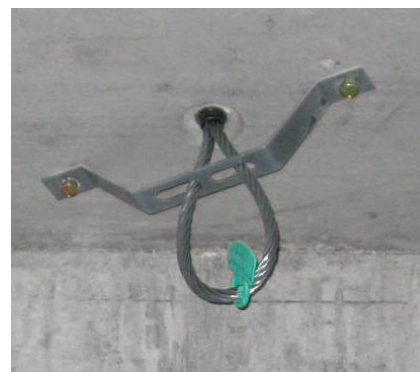
Cable loop installed in a lift shaft
