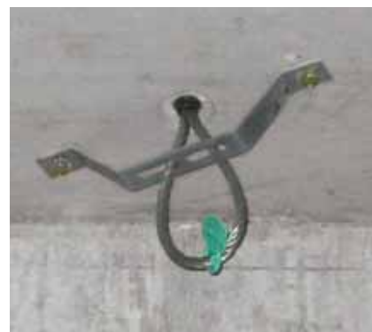
Cable loop installed in a lift head
