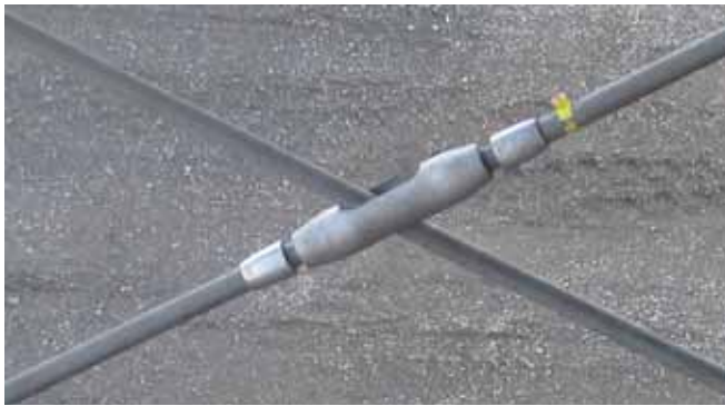
Cross-bracing with a cross-coupler
