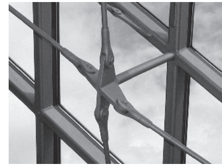
Under-tensioning of glass façade elements with DETAN tension rods
