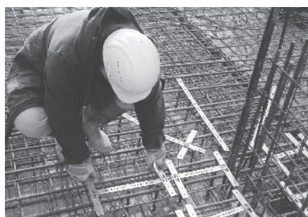
(Above) HDB shear elements are placed after reinforcement work
