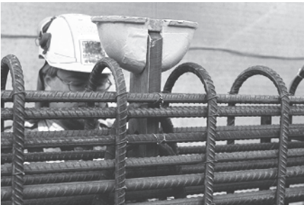
Lifting anchors with recess formers
