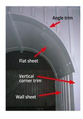
The bottom of the flat white sheets fit behind the jack arch wall sheets. On the joint between the edge of the jack arch ceiling sheets and the main arch wall sheets use the hollow section angle trim which will flex to suit the curve of most jack arches. These are secured with 38mm hex head fixings (AL-TRF38L) through the flat sheet into the AL-CB5025 batten.
