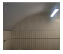
The T & G cladding planks are scribed tight to the arch ceiling sheets – additional capping trim or flashing can be used here if required. Where the planks are not running all the way to the floor they will tuck neatly behind the metal wall sheets.
