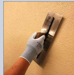
**7.** Cross trowel to ensure the minimum amount of material is applied to the correct thickness.
