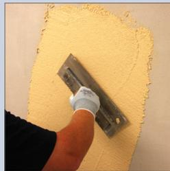
**6.** Apply using a stainless steel trowel or suitable spray equipment.
