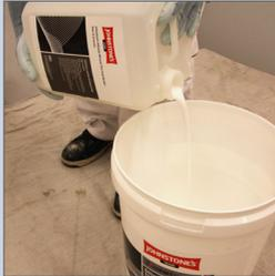
**2.** Thoroughly shake part A and pour it into the mixing tub.
