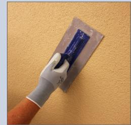
**8.** Finish with a plastic float, working the material in small circular motions.
