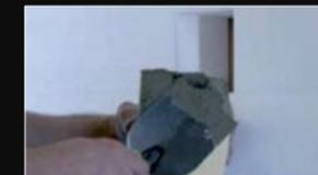
3. Apply Johnstone's Insulation Panel Adhesive to entire back face of Power Block and fix flush
