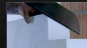
1. Cut EWI system insulation to accommodate power block.
