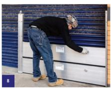
Continue the process of inserting all panels along the entire barrier length, ensuring all bottom panels are lowest, then middle panels, then top panels.
