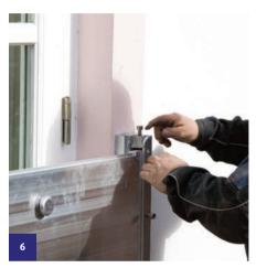
Insert compression block into fixed wall post and finger tighten. Finger tighten the horizontal compression screws by hand, so that panels begin to depress against the rubber seal on the inside of the channels, then finger tighten the vertical compression screws on the top compression blocks by hand, which will depress the rubber seal on the bottom aluminium panel to the floor.
