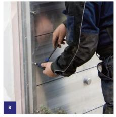
The horizontal screws can now be tightened. DO NOT OVER TIGHTEN.
