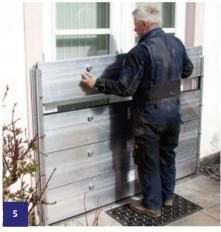
Continue the panel deployment process with the insertion of the intermediary panels (these panels have top seals on only) and are labelled MIDDLE PANEL. Finally add the top panel which has no seal and is labelled TOP PANEL.
