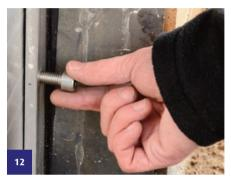
Finger tighten the horizontal compression screws by hand, so that panels begin to depress against the rubber seal on the inside of the channels.
