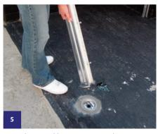
Insert demountable post into ground insert ensuring located correctly (note FRONT indicated) and finger tighten (only) the top securing nut.
