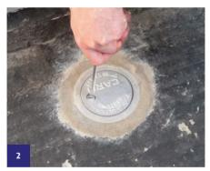
When the threat of flooding becomes apparent, commence the deployment process by unfastening ground insert dust caps with screwdriver or similar.
