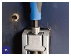
Equally tighten compression blocks in fixed wall posts...
