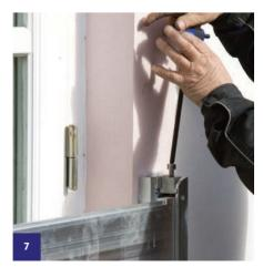
Now equally tighten compression blocks in fixed wall posts.
