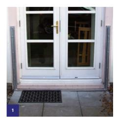
When the barrier is not deployed, the opening remains unobstructed allowing full access to the property. When the threat of flooding becomes apparent, the deployment process can commence.
