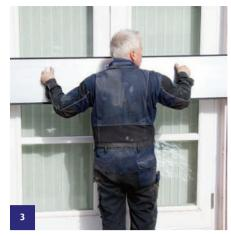
Prior to slotting in the first Aluminium Panel, please ensure that the floor surface and its immediate surroundings are free from any debris. Once this is done, you can start inserting the panels.
