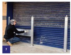
Begin inserting the first panel into the rails, ensuring that you start with the rubber sealing bottom panel first (these panels have seals on both top and bottom).
