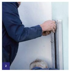
First remove the compression blocks at the top of the rails and unscrew the horizontal fixings, which are positioned down the length of the fixed wall rails. This is to ensure they do not obstruct the deployment of the panels.
