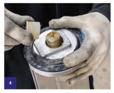
Before inserting the demountable post, please ensure that the post and ground insert are free from any debris.
