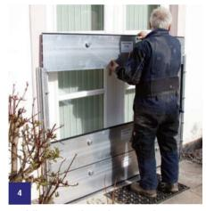
Carefully insert each panel, ensuring that you start with the rubber sealing bottom panel first. These panels have seals on both top and bottom and are labelled BOTTOM PANEL.
