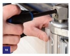
Lightly secure demountable posts by using tool provided – DO NOT TIGHTEN AT THIS STAGE.
