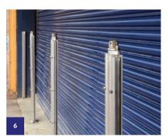
Continue this process along the entire barrier length until all posts are deployed.
