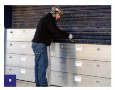
Complete the installation by inserting all panels, ensuring that all middle seals (between panels) are correctly seated and not misplaced.
