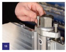
Finger tighten the vertical compression screws on the top locking block by hand, which will depress the rubber seal on the bottom aluminium panel to the floor.
