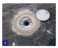
Once the caps have been loosened across the entire barrier length, lift the caps out to prepare each insert for deployment of demountable post.
