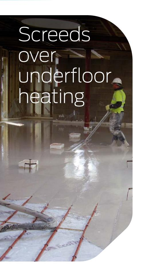
When screed is installed over underfloor heating, the screed has to be of suitable depth - both for strength and to provide sufficient cover over the underfloor heating pipework.
