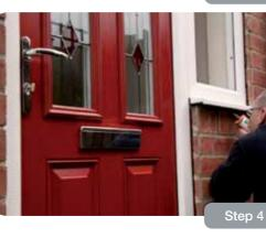
Remove all protective films on the outer frame profiles as soon as the installation is finished and prior to perimeter sealing.
