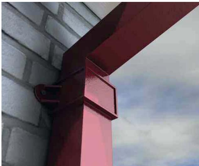
Heritage square and rectangular pipes are available in 3 pipe sizes and 3 pipe lengths, together with a complete range of fittings. A spigot and socket system, which can be finished to replicate cast iron or with BBA certificated powder coatings in a choice of colours. Complementary rainwater heads available to suit.
