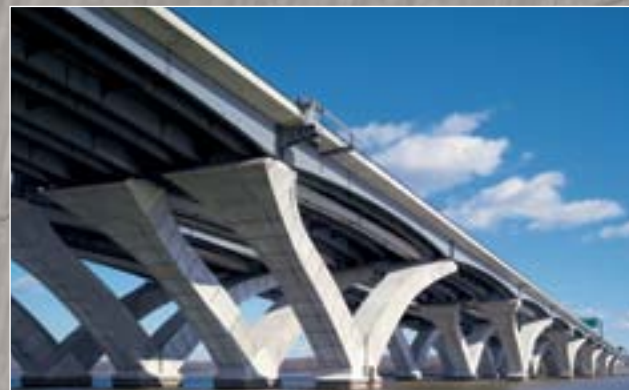
Woodrow Wilson Bridge, Washington, USA
