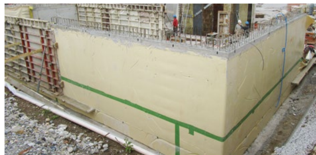
Open excavation with SikaProof®-A – after removing the formwork the anchor penetrations have to be sealed.
