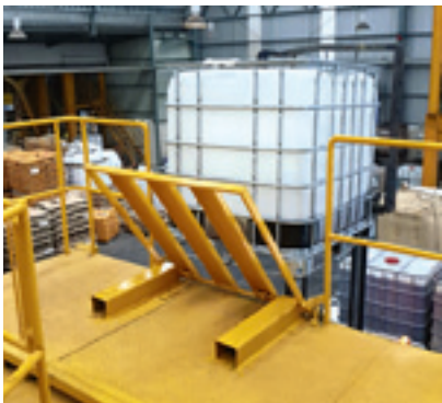
AUTOMATIC SAFETY LOADING GATE FOR WORKING PLATFORM, SIKA INDONESIA PLANT SURABAYA, INDONESIA
