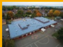
LIQUID APPLIED ROOFING
