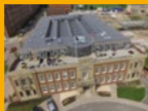
SINGLE PLY ROOFING
