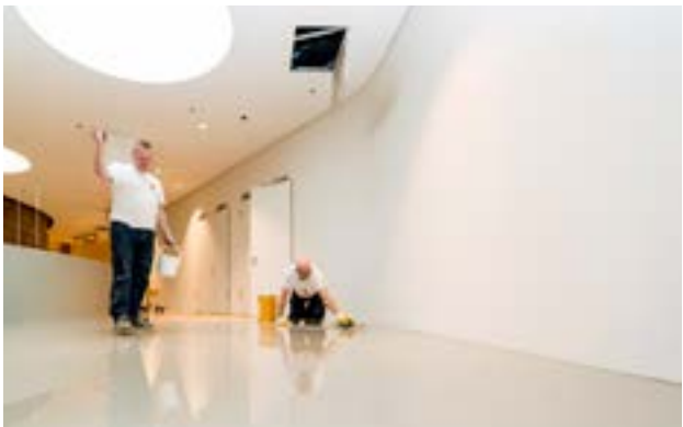
STEP 4. A wide selection of liquid resin products is available in an almost unlimited amount of colours to address many types of use. Decorative flakes or anti-slip aggregates may be broadcasted into the wet surface.
