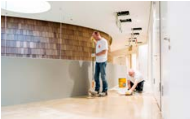
STEP 2. A liquid primer is applied to assure good bonding of the flooring, which is typically done by trowel and roller. The adequate method can be selected depending on the quality of the subfloor.
