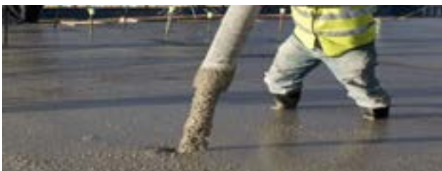
Pumped Concrete
