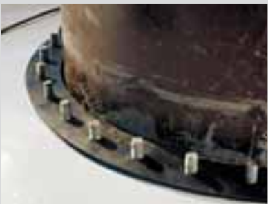
Loose- Flange construction in case of water pressure
