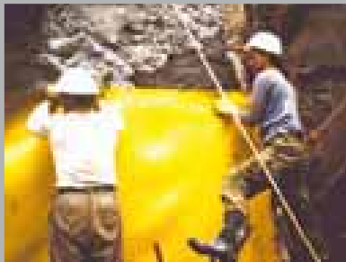
Ignoring substrate requirements and omitting protective backing materials
