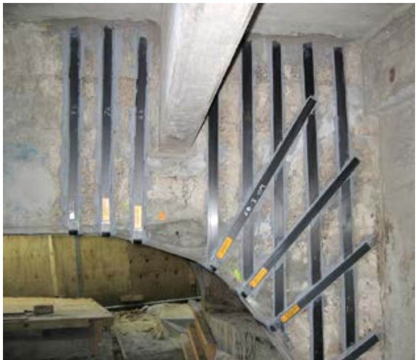
Sika® Carbodur® strips and CarboShear L plates bonded to the concrete structure.
