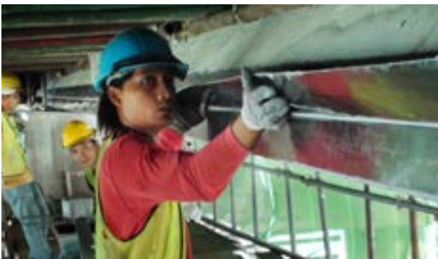
Installation CarboDur®
