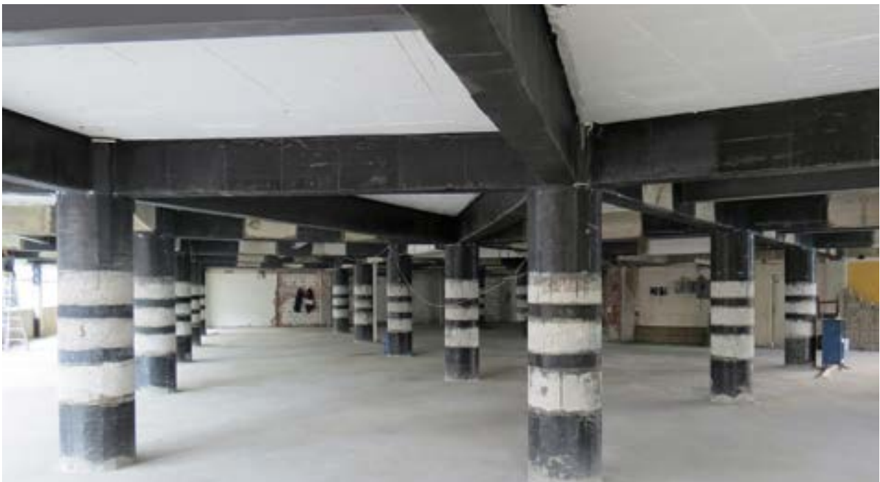
Beams and columns strengthened with SikaWrap®
