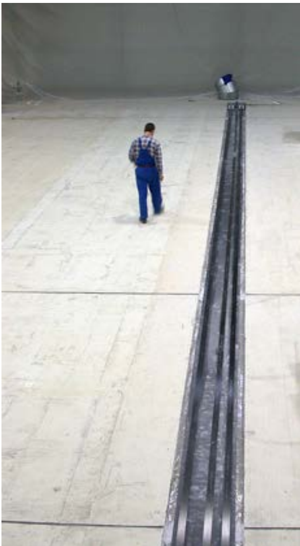
The longest post-tensioned CFRP-plates ever installed
