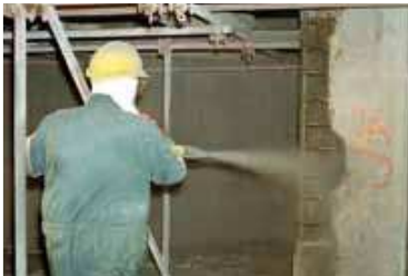
Machine applied concrete repairs
