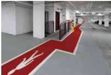
Flooring in car parking areas
