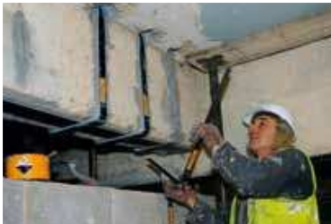
Shear strengthening of beams
