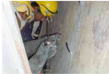
Watertight crack sealing by injection
