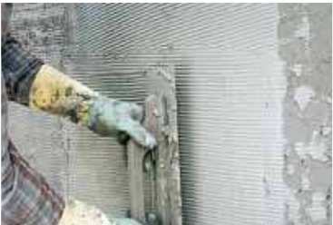
Hand applied mortar
