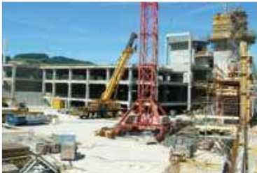
Site batched concrete production
