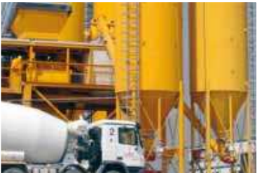
Ready-mix concrete production
