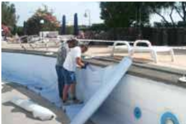
Waterproofing with flexible Sikaplan
