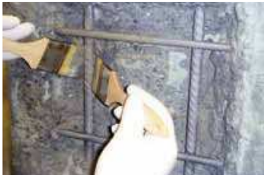
Protection of steel reinforcement
