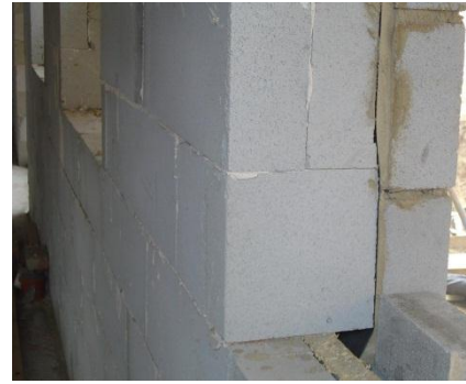
Reveals can be formed from cut Airtec blocks with a slip plane of dpc placed at the interface with the outer leaf
