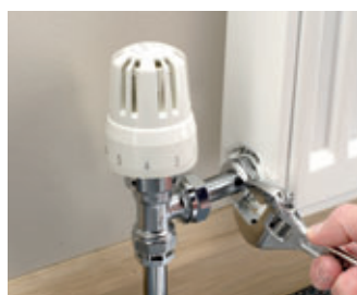
2. The tailpiece is tightened into the radiator.
