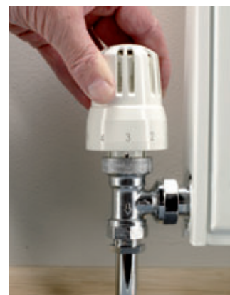
4. The head is pushed down, locking it into place.
