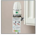
Once installed the user information tag is placed around the collar beneath the TRV to help the user.
